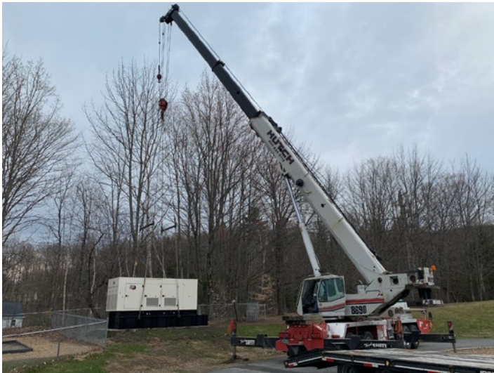
(Hutch Crane Service helped with the installation of the new generator.)
